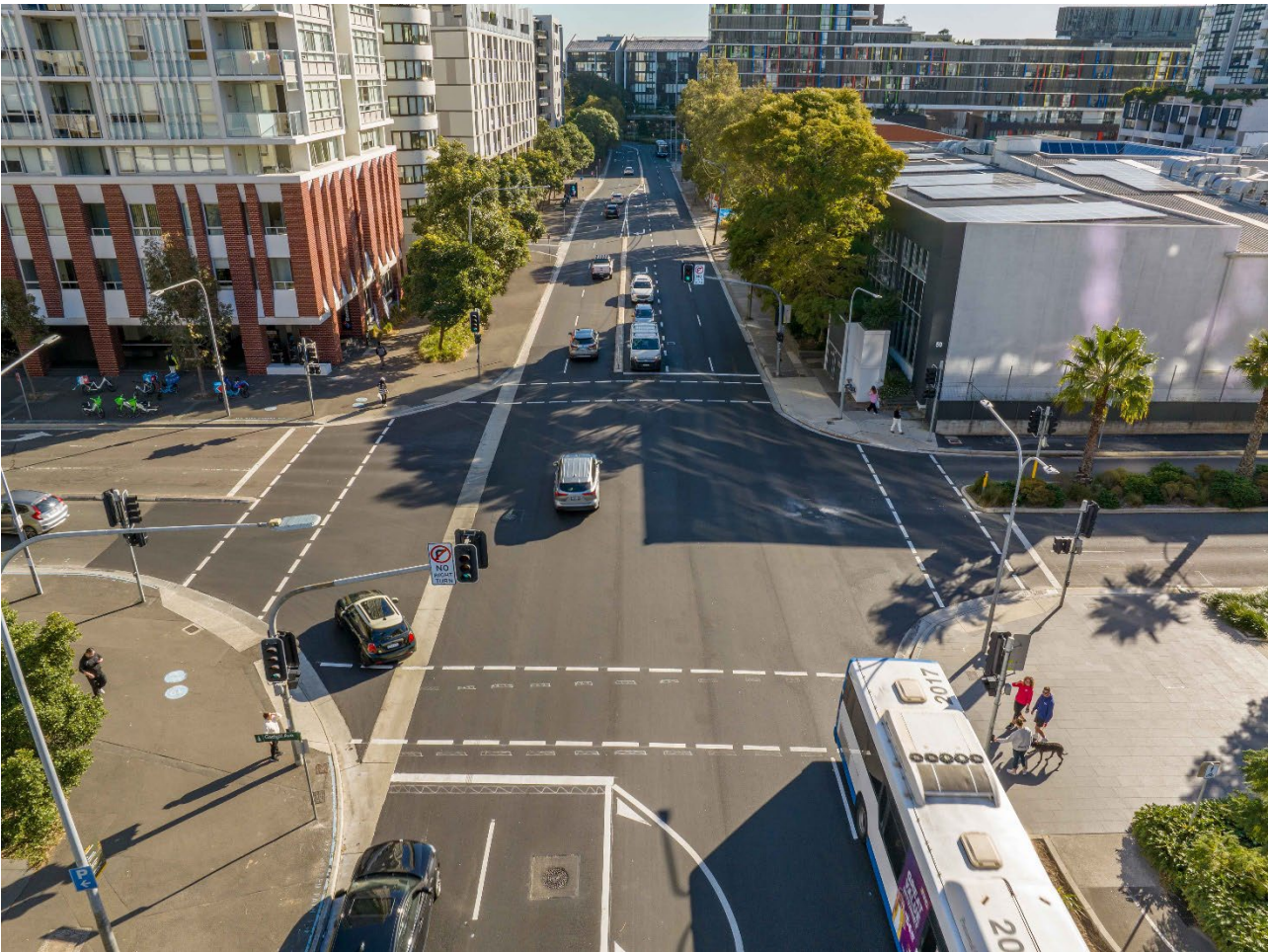
O'Dea Avenue's renewed road surface (Photo by Sydney Civil)
